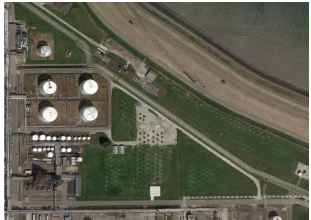
Figure 1. Phytoremediation at Terneuzen
